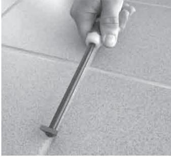
**Step 2.1.** If not done so already, carefully remove the tile/stone/marble floor covering over the damaged cable area. Removal of the grout around the affected tile(s) must be done with a blunt instrument such as a hand-held grout-removal tool. **DO NOT USE A KNIFE!** Gently break out the tile with a small hammer, removing the fragments as the tile is broken up.
