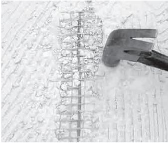
**Step 2.2.** Remove enough mortar and tile to expose about **4" to 5" of free wire on both sides of the damaged portion.** Part of the wire may be visible so that the mortar can be removed carefully around the damaged wire using the hammer and/or chisel. Mesh can be cut with scissors in order to free the wire.
