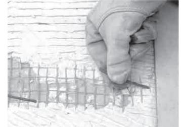
**Step 4.5.** Use a glove or other protective cloth to pull off the loosened jacket slug. Do not touch the hot jacket slug with bare fingers. The slug will be very hot and will burn!
